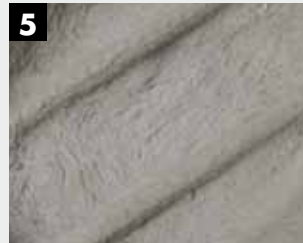
5 Prewet the broken away surfaces and then vigorously brush in KEIM Concretal-MKH as bonding bridge.
