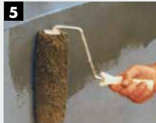
5 Apply two protective coats of KEIM Concretal-W a) diluted priming coat b) undiluted finishing coat in each case applied by brush, roller or airless sprayer
