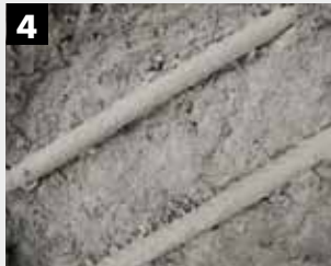
4 Apply two protective coats of KEIM Concretal-MKH to the derusted reinforcement, allowing at least 3 hours to elapse between coats. Apply first coat immediately after rust removal.
