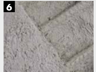
6 Fill defective areas with mineral KEIM Concretal-Mörtel-R in the moist bonding bridge. Layer thicknesses of 0.5–5 cm are possible, multiple layers must be used from a thickness of approx. 2.5 cm.
